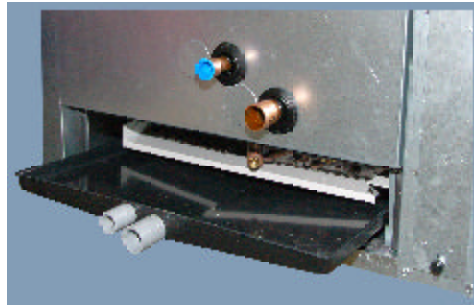
Figure 2 - Drain Pan with access door removed
